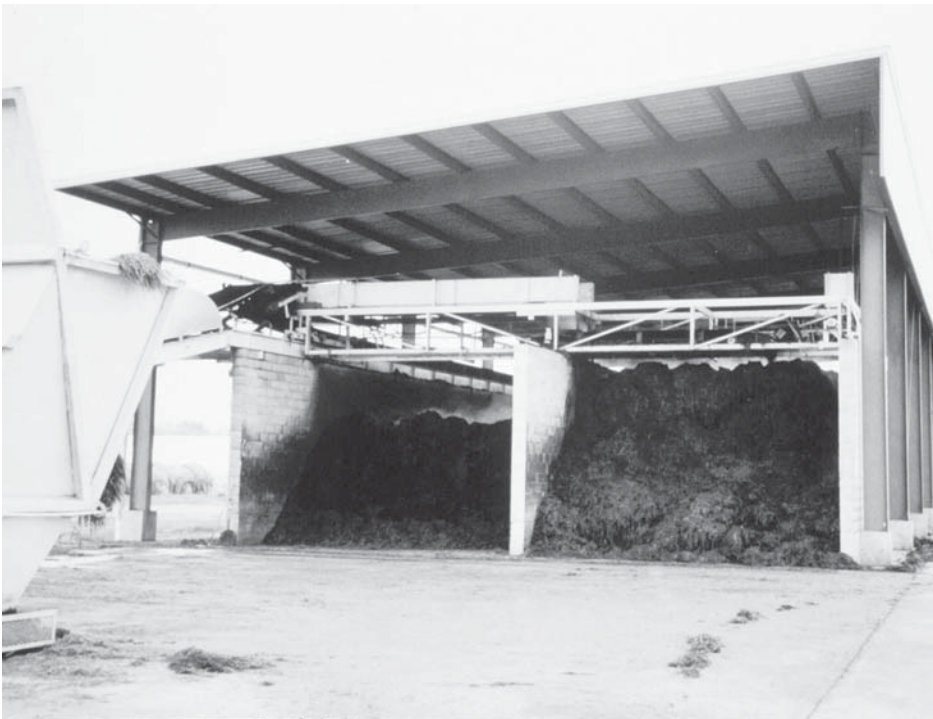
Figure 4. This aerated substrate preparation system has a piped concrete floor under the substrate that forces air through the substrate to maintain aerobic conditions during the composting process.
